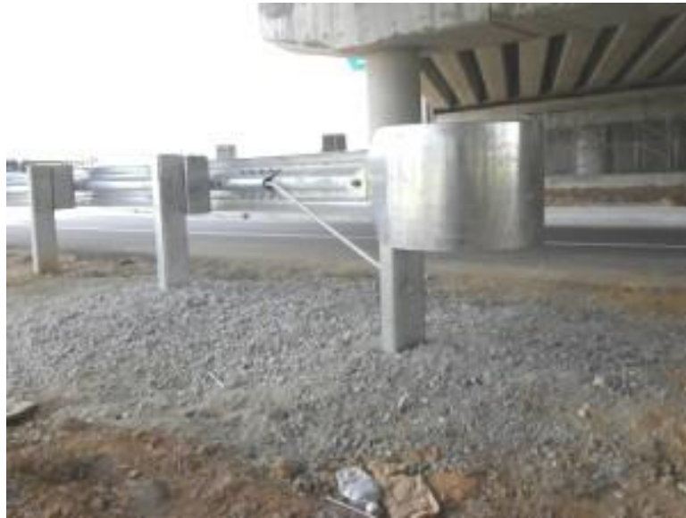
Rajah 47 : Terminal Anchorage Unit
