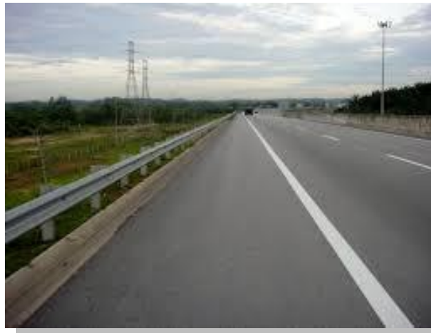
Rajah 14 : Shoulder paved / berturap
