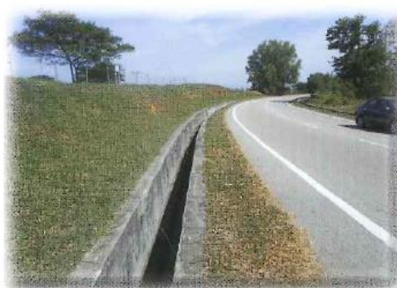
Rajah 50 : Roadside Drain
