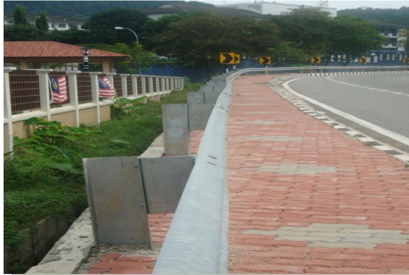
Rajah 19 : Unpaved Interlocking Shoulder
