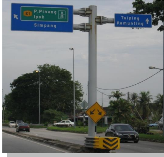
Rajah 37 : Tiang papan tanda jenis gantry.
