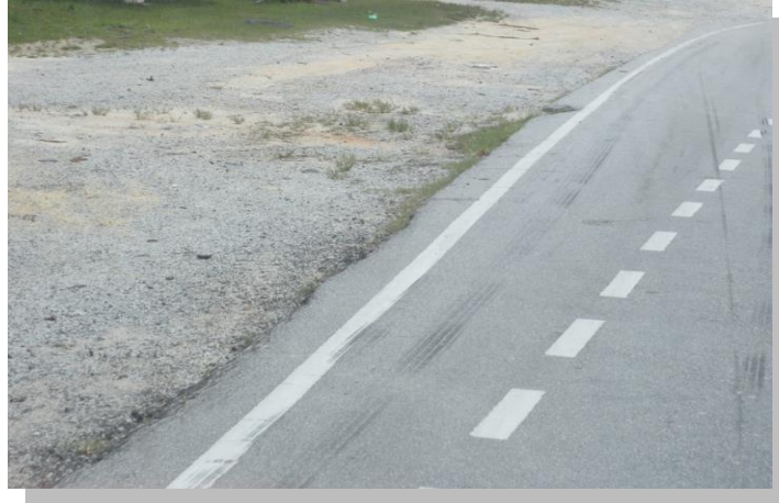
Rajah 17 : Unpaved Gravel Shoulder
